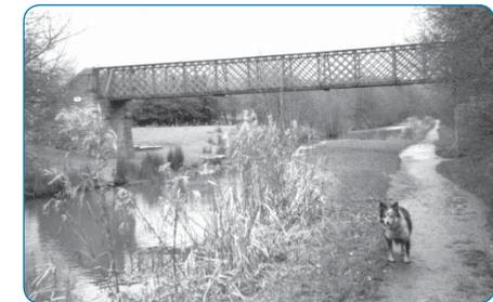
**i** The bridge was originally built for pedestrians with Hagg swing bridge below for cattle and vehicles. The site of the swing bridge is overgrown but clearly visible.
